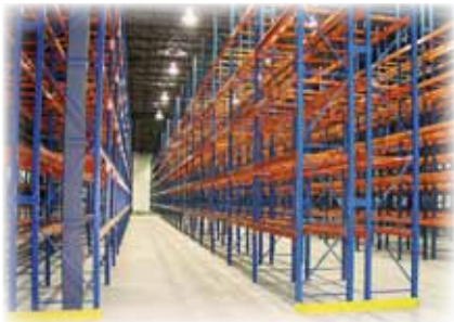
NORTH AMERICAN RACK
